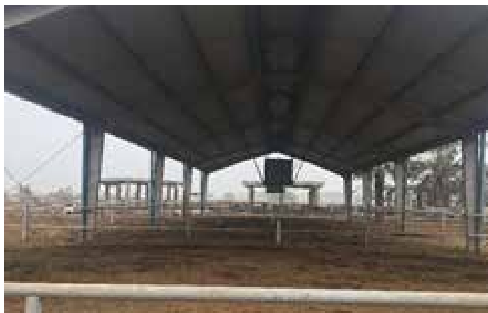
Figure 4 Steel structural shed, Deda Research & Development Farm, Kasur, Pakistan.
