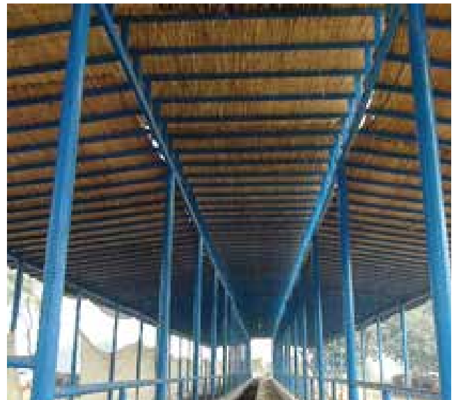
Figure 2. Steel pipe with thatch roofing, Nawab Nadeem-ud-din farm, Multan.
