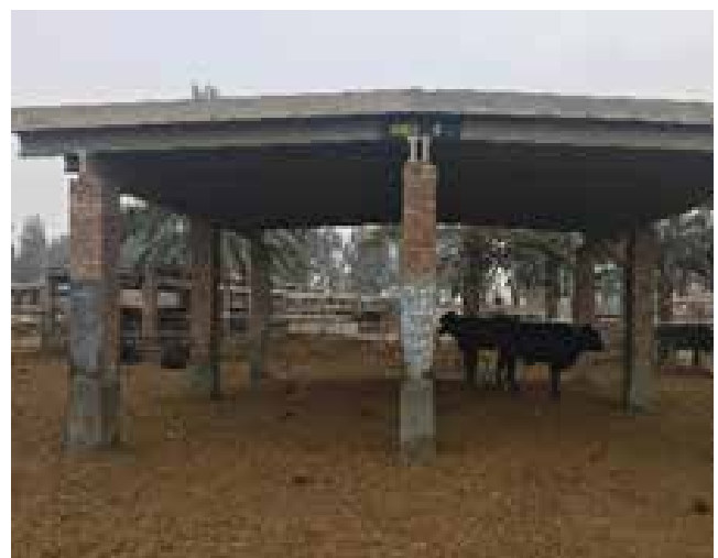
Figure 3. Precast roofing with brick masonry, Deda Research & Development Farm, Kasur, Pakistan.
